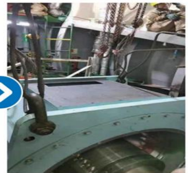
Installation of upper part of stator
