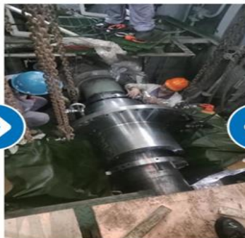
Installation of expansion sleeve
