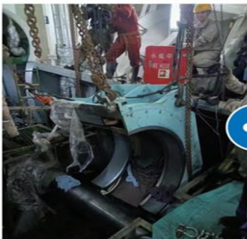
Lower half of stator lifting
